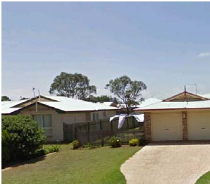
Figure 3: New suburban houses, Toowoomba, Queensland.
